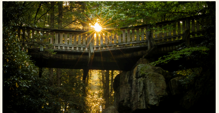
Bridge Over Elakala Falls No. 1
